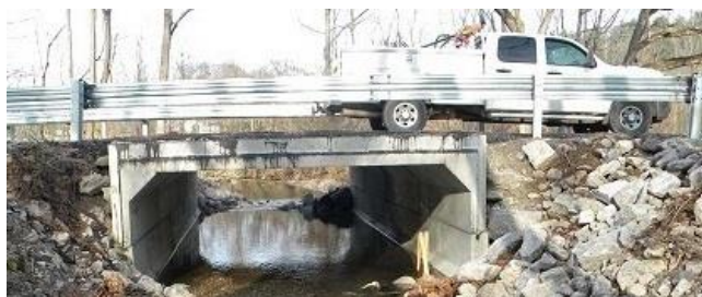
Finished construction of 12' x 5' box beam culvert.
