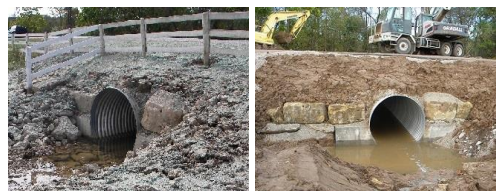
Views of finished replacement culvert.
