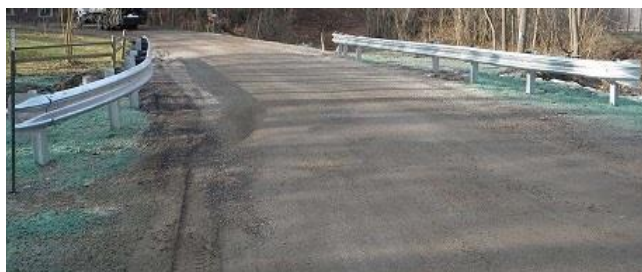
New roadway is now 22' face to face guardrail.
