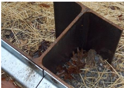
Top view of steel column set into bedrock.
