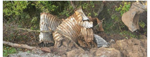
Removal of existing damaged culvert.
