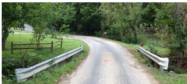
Old roadway with 12' face to face guardrail.
