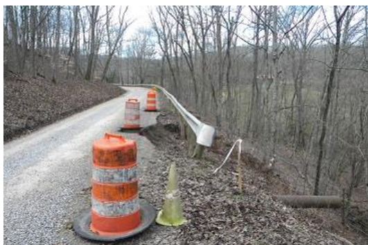
View of the deteriorating roadway surface and slip.
