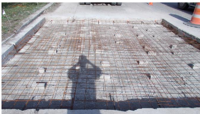
Roadway repair prepped for pouring.
