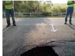
Sinkhole formation due to culvert failure.
