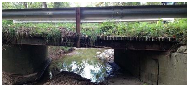
Deteriorated wood deck and crack in abutment.
