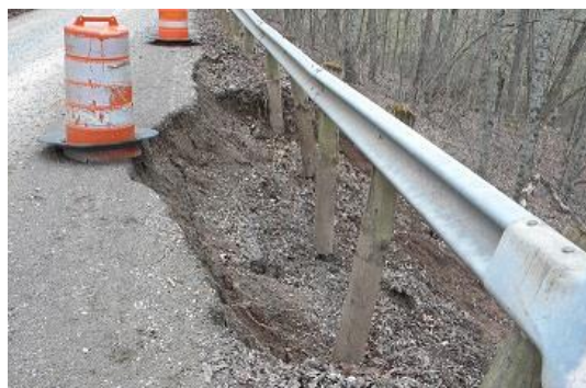
Closer view of the slip and eroding roadway surface.
