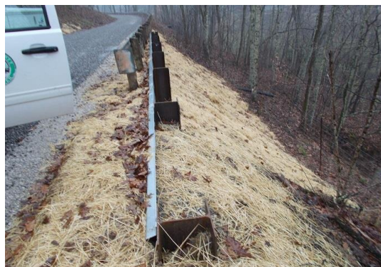
Finished construction of drilled pier wall.
