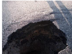
Sinkhole formation due to culvert failure.
