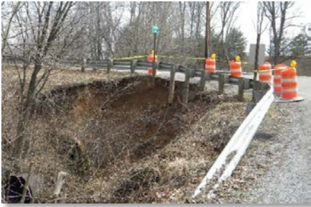
Culvert failure on CR 110.
