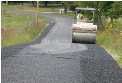
Compacting the road surface.
