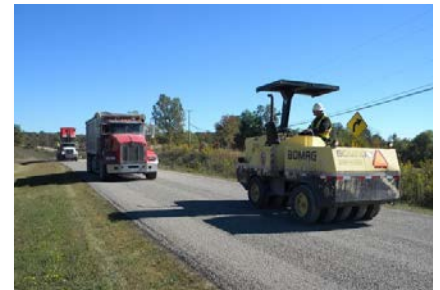
Final stages of chip seal.
