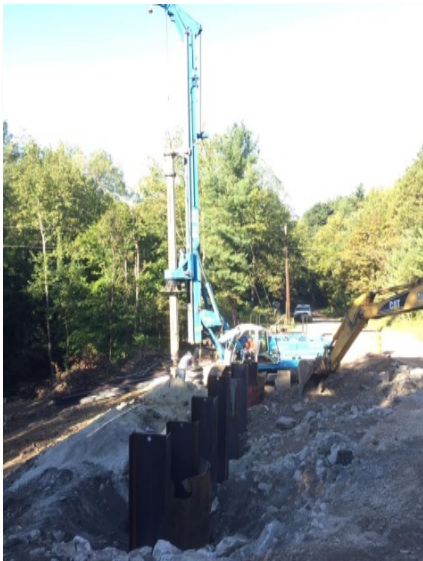
Pier wall drilling.
