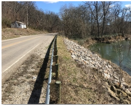
Slope reconstruction and guardrail complete.
