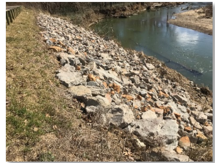
View of completed rock channel protection.
