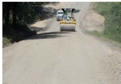
Compacting the road surface on CR 20.
