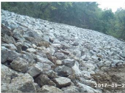
Rock Channel Protection complete
