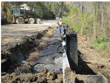
CR20-5.27 Bev Sargent inspecting drilled Pier Wall construction
